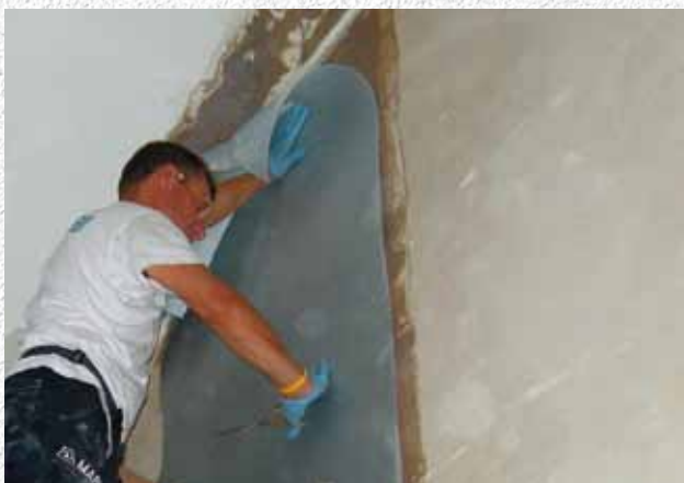
Application of MapeWrap EQ System . A. Pio Middle School. Carpi, Modena.
