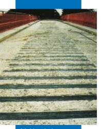
A bridge-deck reinforced with Carboplate
