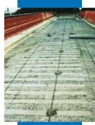
Carboplate covered with Mapegrout BM
